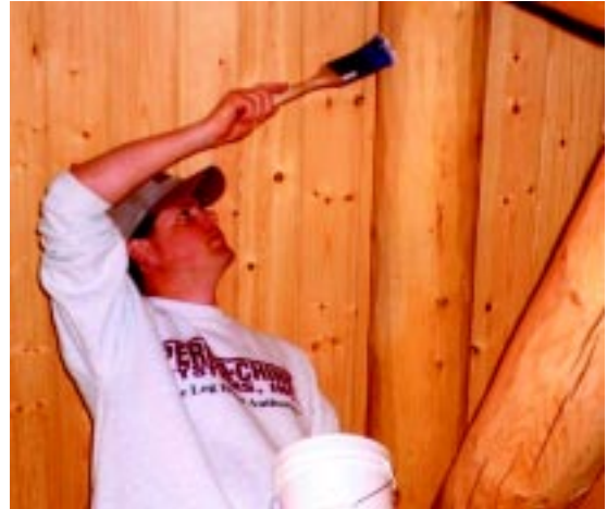
Application of Acrylic Gloss finish for interior log wall
